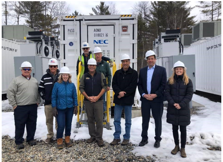
MEW staff pose with State Senator Brad Farrin and New England Battery Storage partners in front of the storage facilities at the Jones Street substation.
